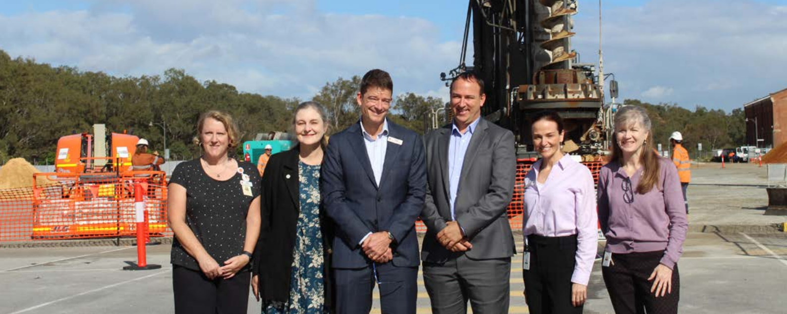
Work commences on the construction of the new St John of God Midland Private Hospital
