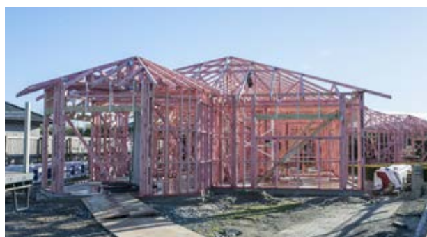
Construction of a second supported-living shared home for adults living with a physical and/or neurological disability has commenced at Selwyn.
