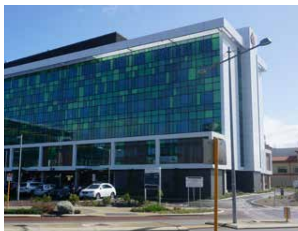
▲ St John of God Murdoch Hospital opened the 120-bed South Wing in July 2014, which is also home to a new 20-chair cancer centre.
