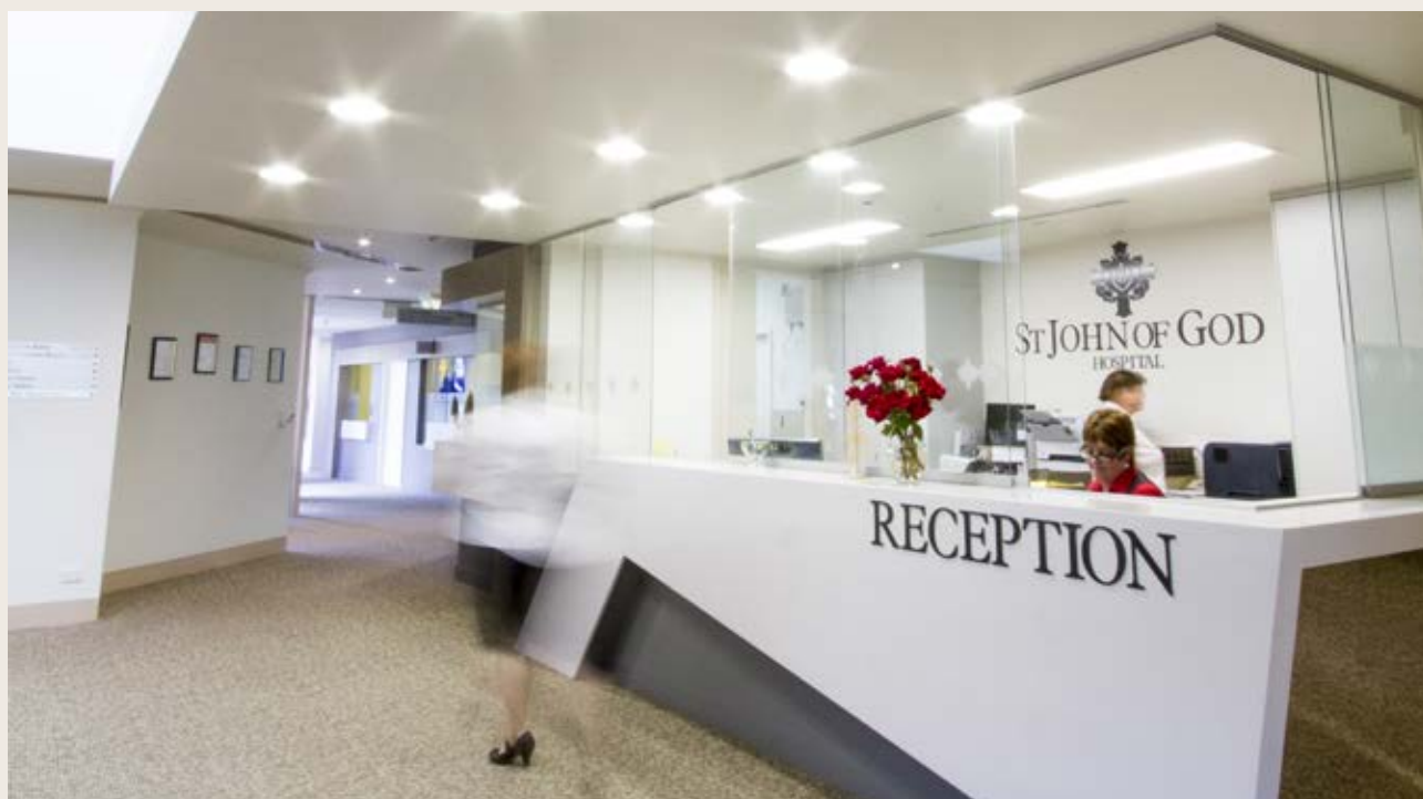
New energy-efficient lighting at our Warrnambool hospital
