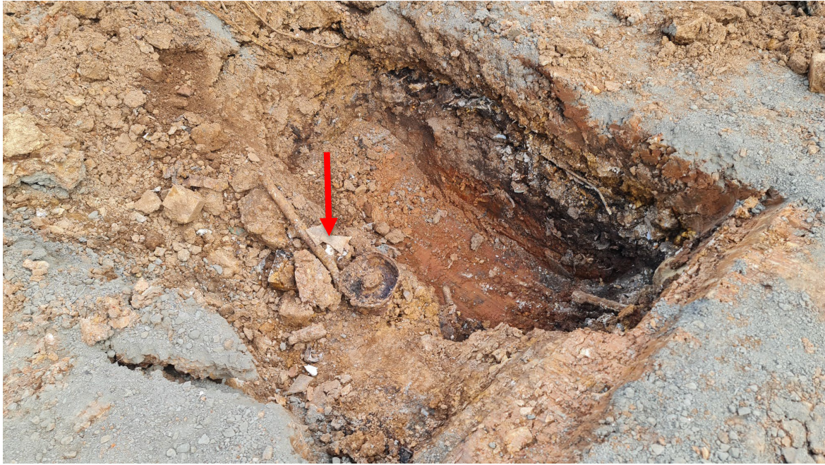
Fill soil in former tennis court area containing metal, glass and pieces of asbestos cement sheet debris. Arrow indicates asbestos cement sheet debris
