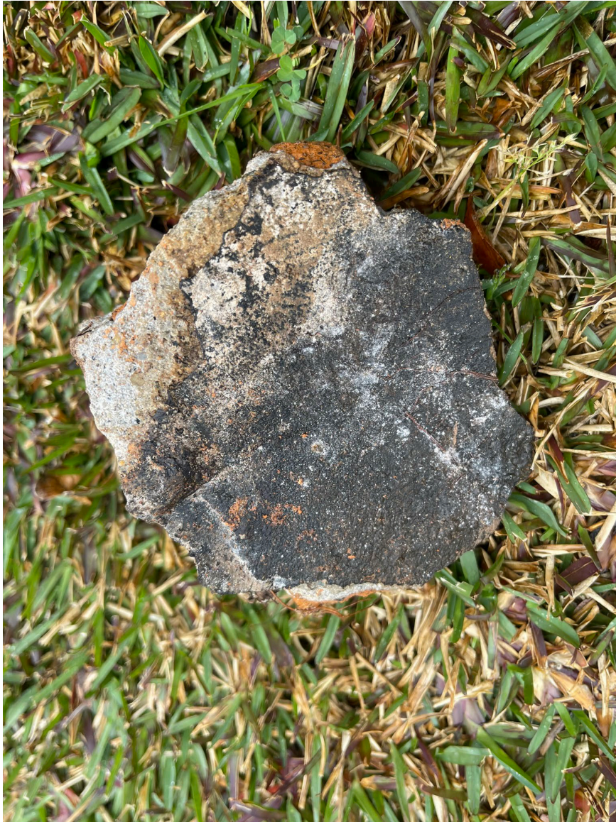
Bitumen waterproofing paint on brick from in-ground water storage tank in the area where the Medical Centre building was located. This material was analysed and found to be free of asbestos
