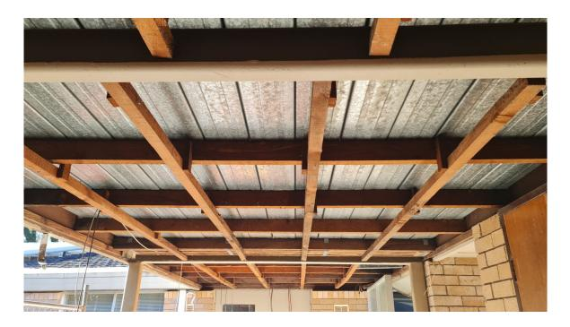
Timber framing to the covered walkway extending between the CTC Building and Belmont House at St John of God Richmond Hospital, 177 Grose Vale Road, North Richmond NSW at completion of visual clearance inspection on 24 August 2022
