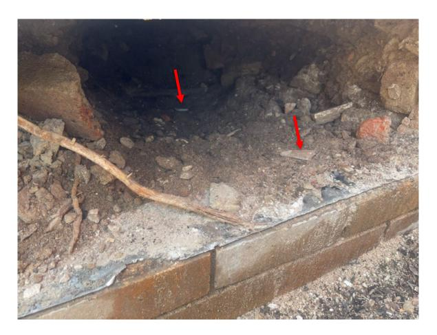
Asbestos cement sheet debris in fill soil below the link bridge between the CTC Building and Belmont House. The asbestos cement debris in this area contains chrysotile asbestos and amosite asbestos
