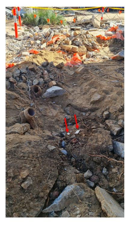
Asbestos contaminated concrete and soil in the area of the former store room (mortuary) adjacent to the CTC building.
