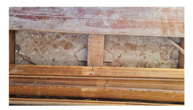
Asbestos cement packing piece between timber floor joist and concrete floor in the upper level of the Monastery Building. This material contains chrysotile asbestos
