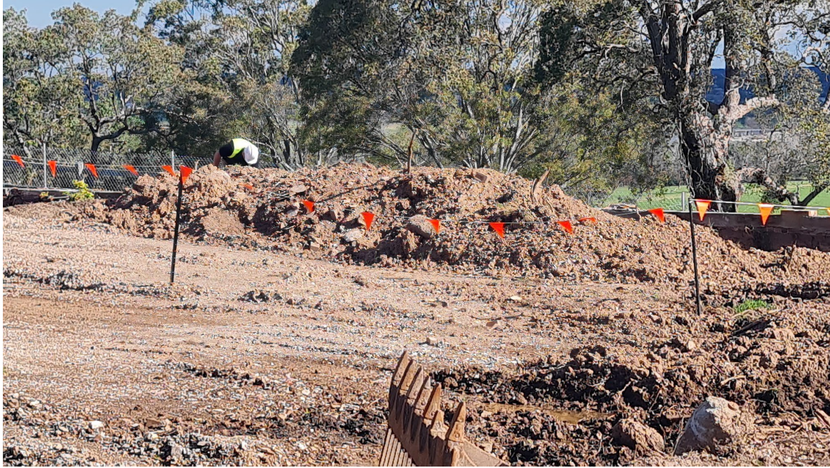
Photograph No. 13 Sandy clay fill soil stockpiled in the rear area of the former monastery building
